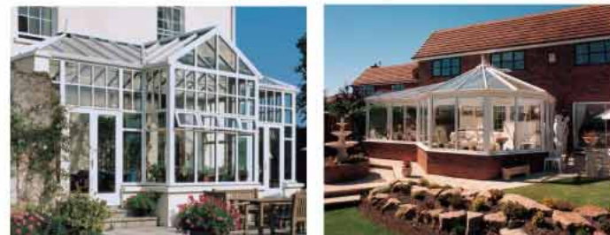
Above Left: T-Style Edwardian with Elizabethan gable front and extended lites. Above Right: This P-shape Victorian is a beautiful addition to this modest home which is eloquently landscaped.
